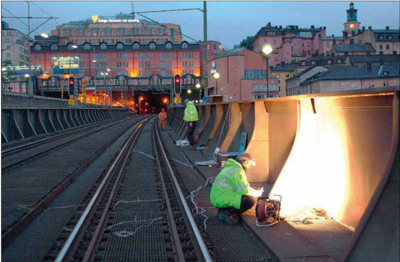
Instrumentation of bridge across Söderström for long time monitoring with accelerometers and strain gauges.
